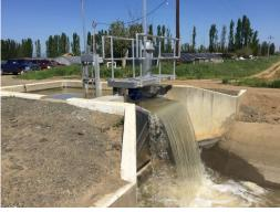
available to us. This last week the engineers were filling it with water and testing the new automatic gates and controllers. This will enable the canal to be controlled much more precisely, minimizing waste water. Up to 175 cubic feet per second can move along. We can
